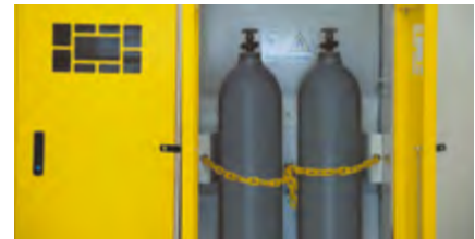
Plastic chain for fixing cylinders
