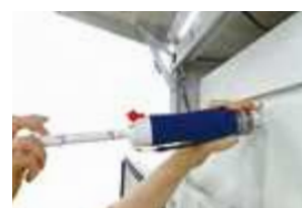
Checking filter saturation
